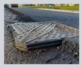
Once Clicklift has been installed, re-place the cover into the now heightened frame.
