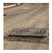
Covers are installed level with the final surface layer removing the need for re-install
