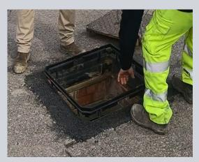
Once aligned, use a rubber mallet to firmly ensure that Clicklift is in place.
