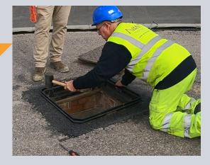
Firstly, remove the cover and line up Clicklift with the existing frame.
