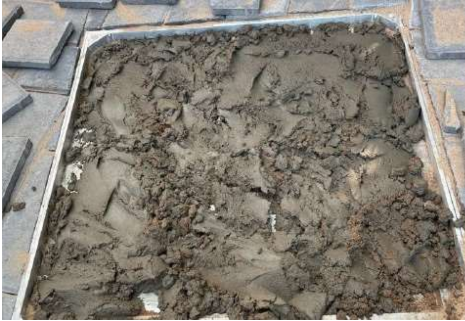
Fig 13 – External paving set directly on mortar bed.
