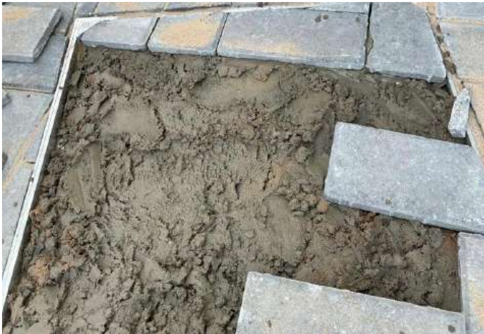
Fig 12 – External installation with fresh mortar bed.
