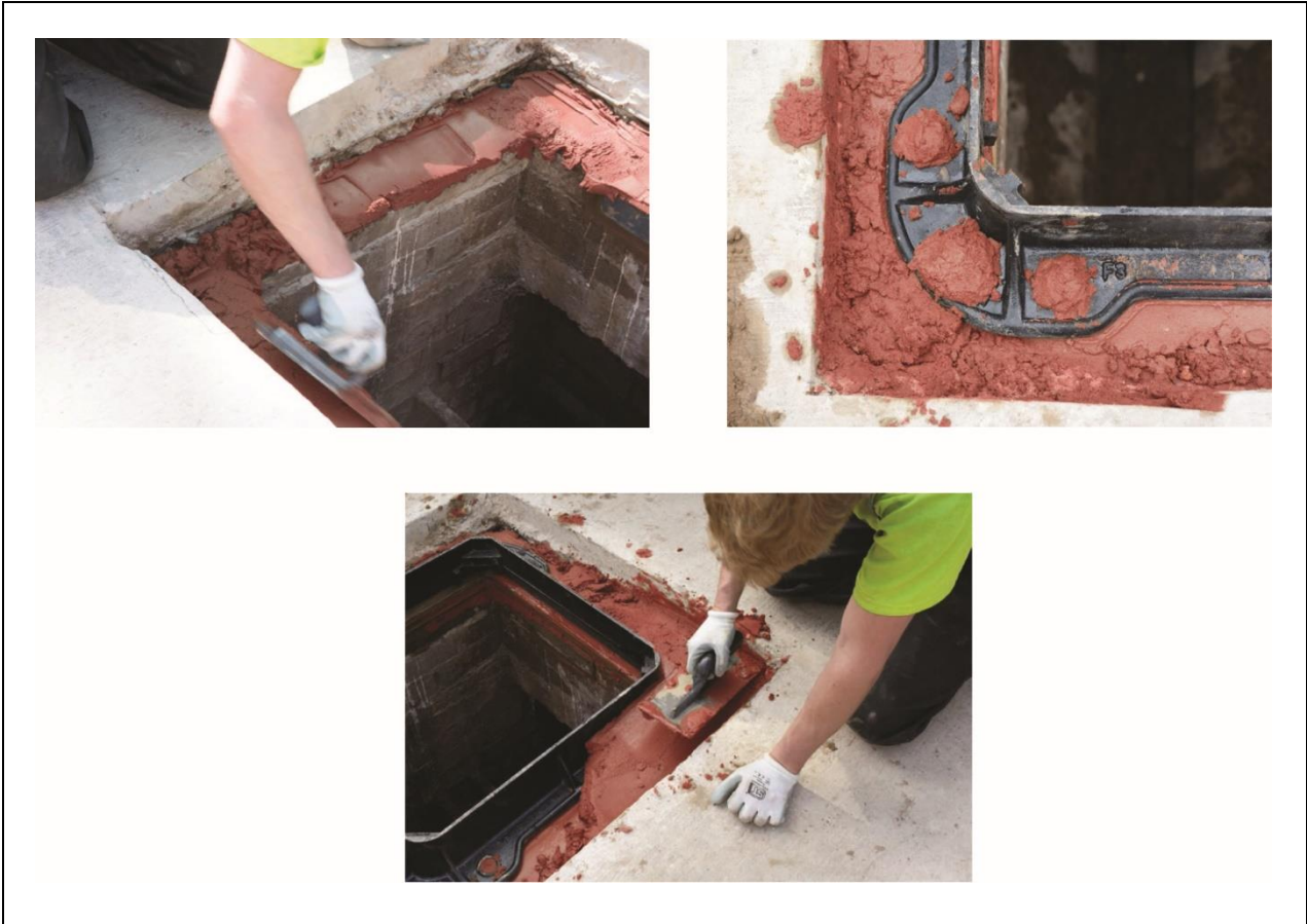
Figure 1 Preparation of damaged ironwork
